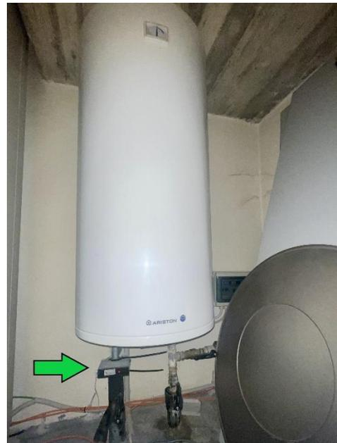
Figura 4: HydroFLOW K40 – Circuito ACS piano -1
